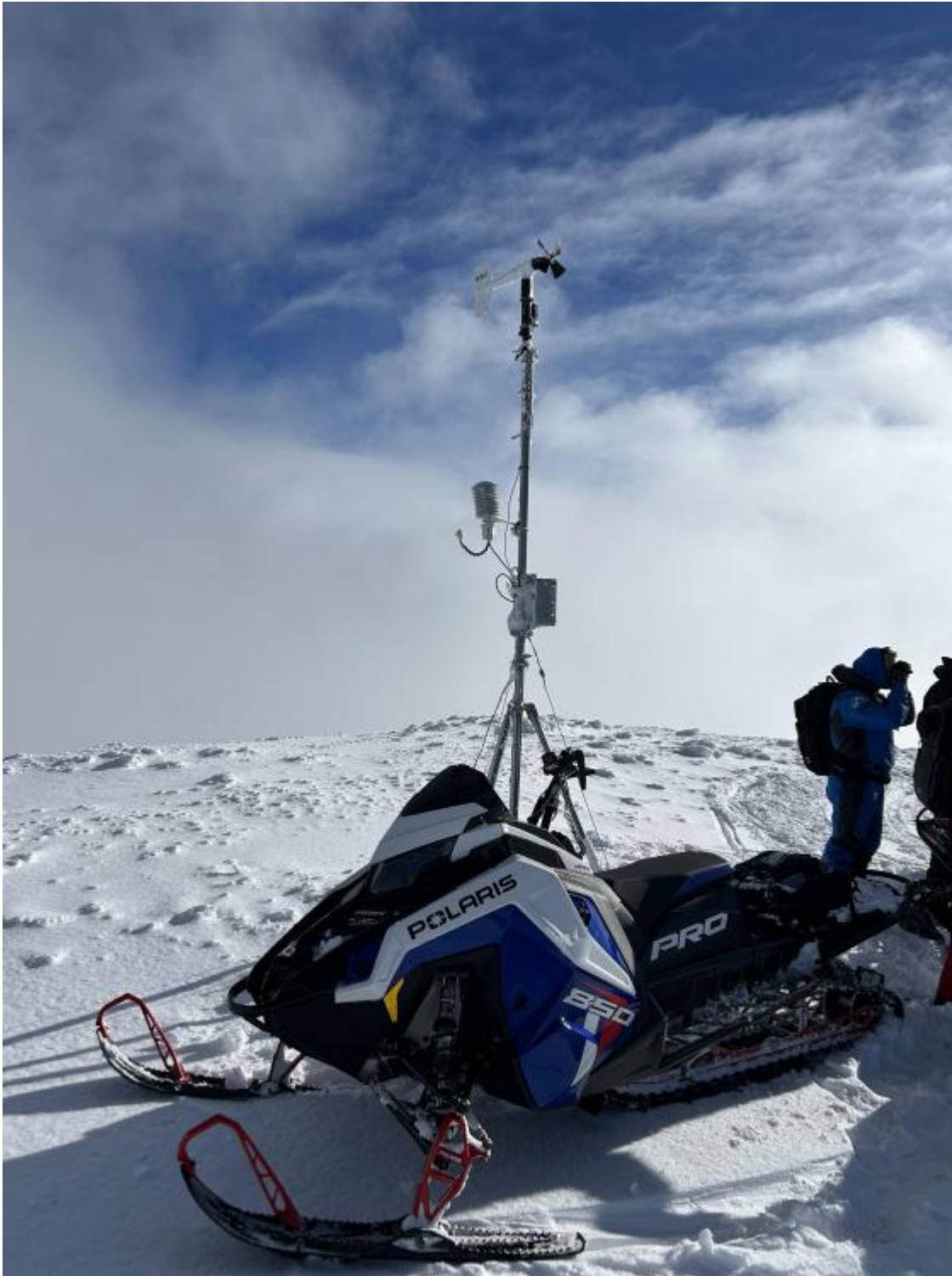
De-iced Sawtell anemometer
