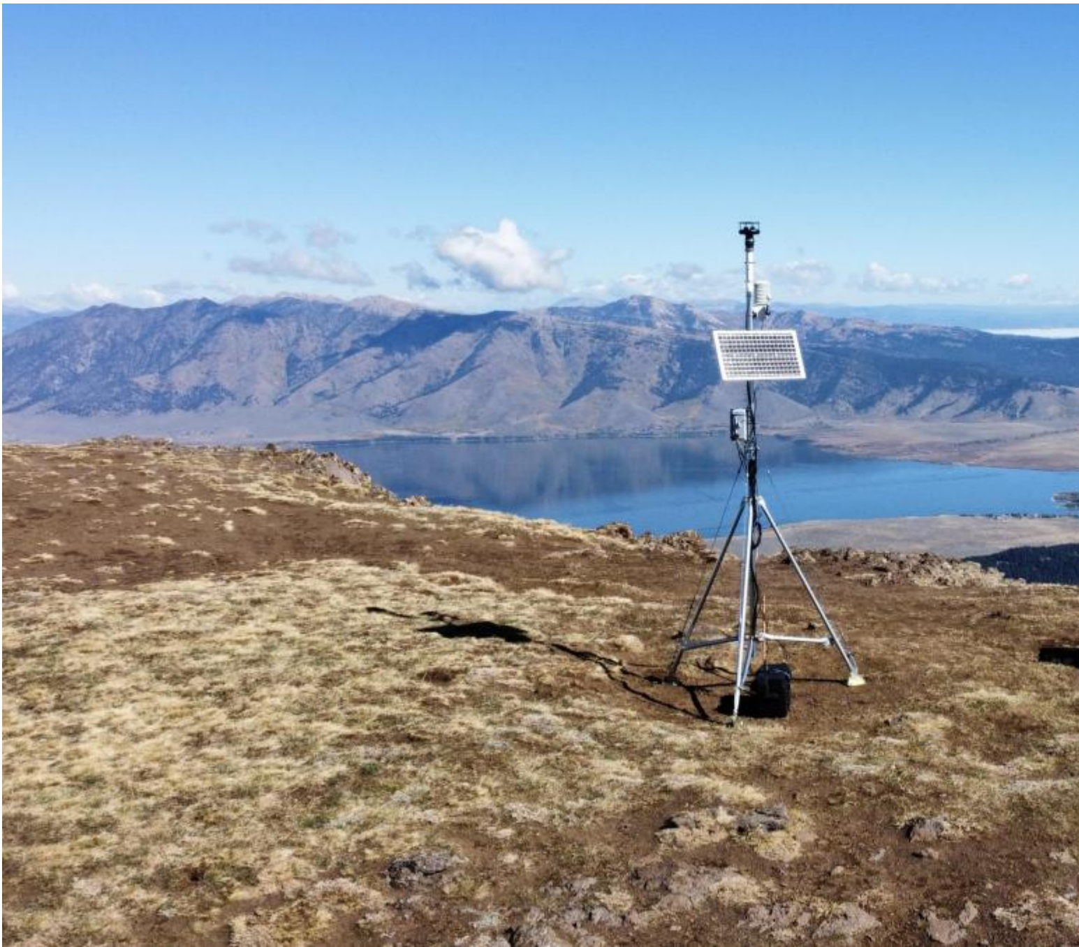
The newly installed Sawtelle Peak weather station. Photo: GNFAC (10/4/2022)
