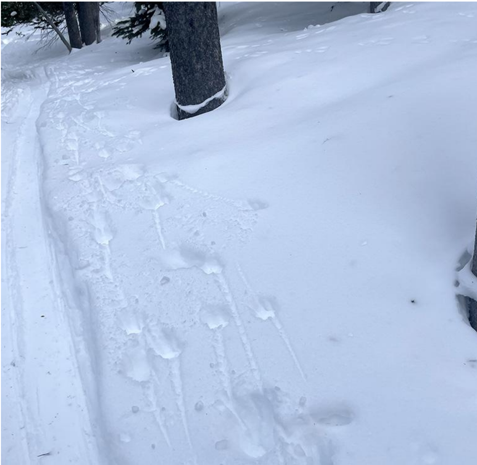
Settlement rings around the base of trees near Cooke City, January 15, 2022. Photo: B. Fredlund
